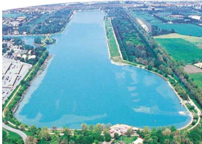
Fig. 4-1 : General view of Idroscalo
