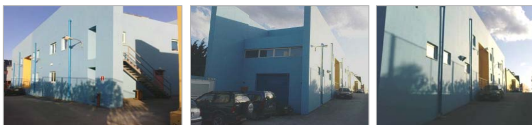
Fig. 3-2: Views of the building.
